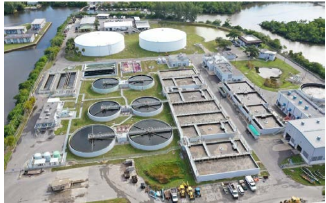
Naples Wastewater Treatment Plant
