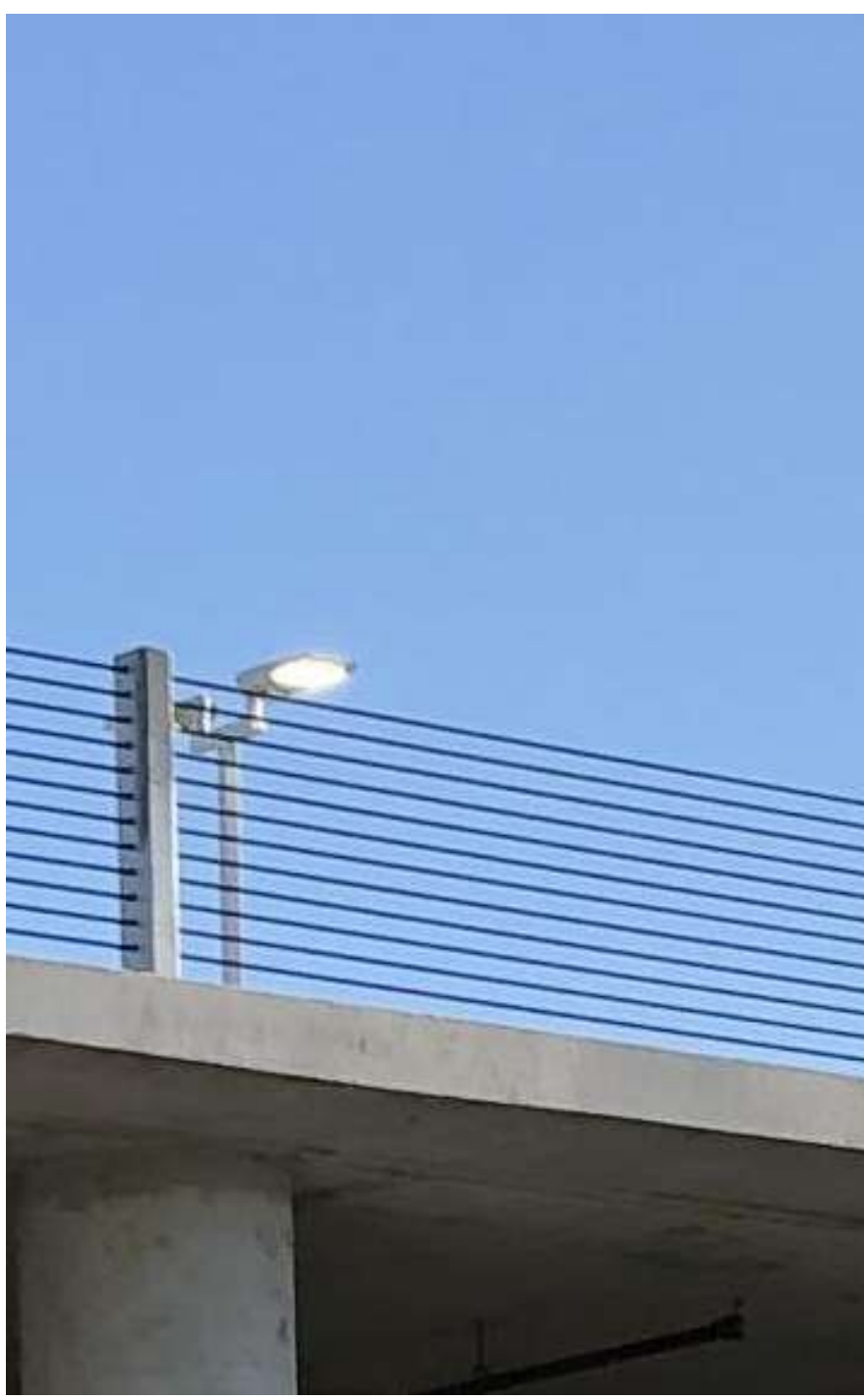
CONCRETE DECK WITH CABLE RAIL
