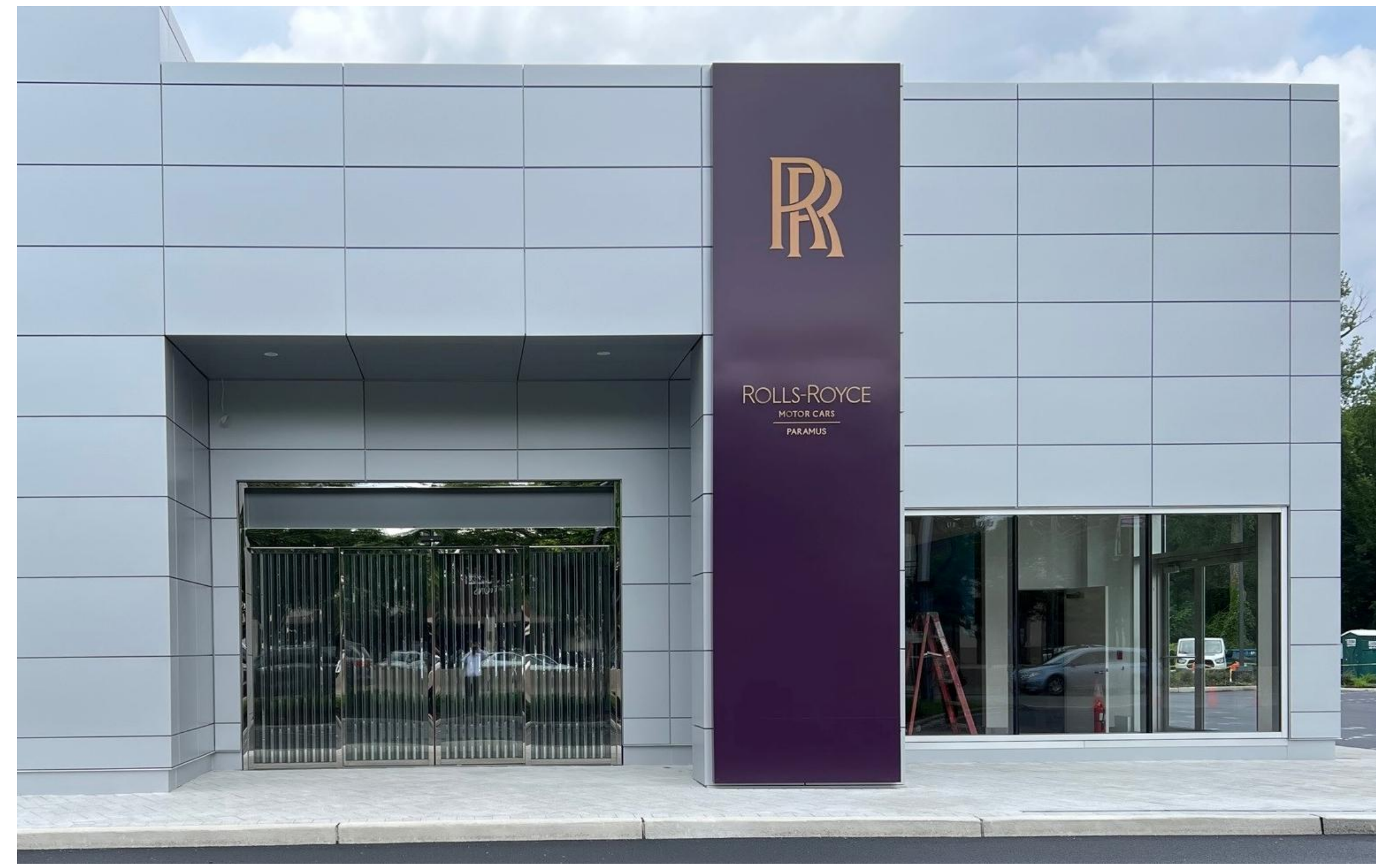
ACM PANELS: ROLLS-ROYCE STEEL (METALLIC SILVER) POWDER COATED STEEL (SIGN): ROLLS-ROYCE PURPLE SPIRIT (RAL 320 20 15) LOGO AND TEXT ROSE GOLD
