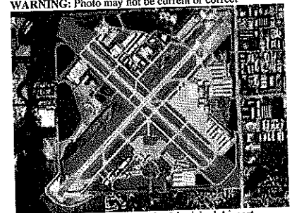
Photo courtesy of Naples Municipal Airport Taken in the Spring of 2014
