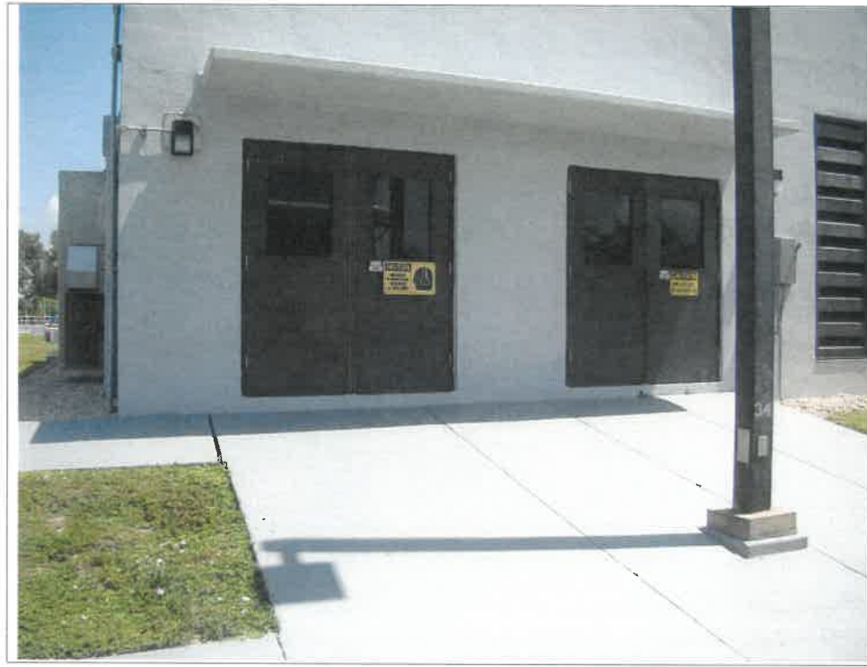
ENTRANCE AND EQUIPMENT ACCESS ELECTRICAL ROOM #1
