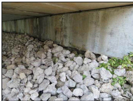
Slope protection at End Bent 1
