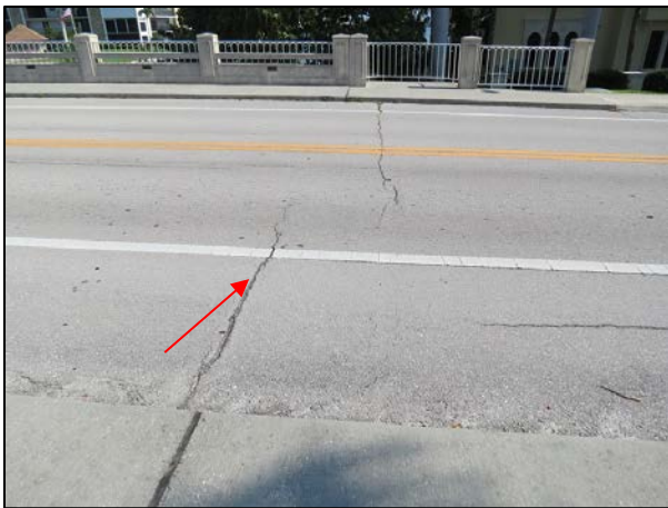
Covered expansion joint at Bent 4
