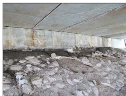
Slope protection at End Bent 4
