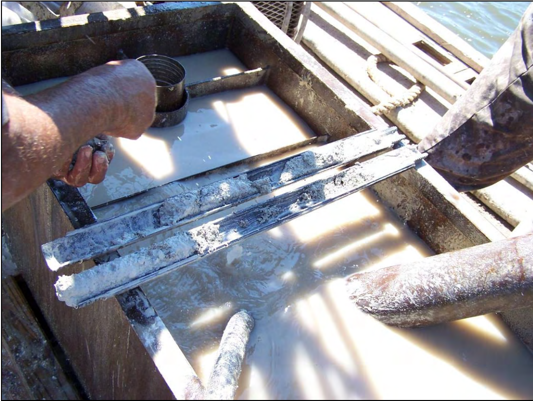
Split spoon recovery from rock boring depth of 8ft to 10ft
