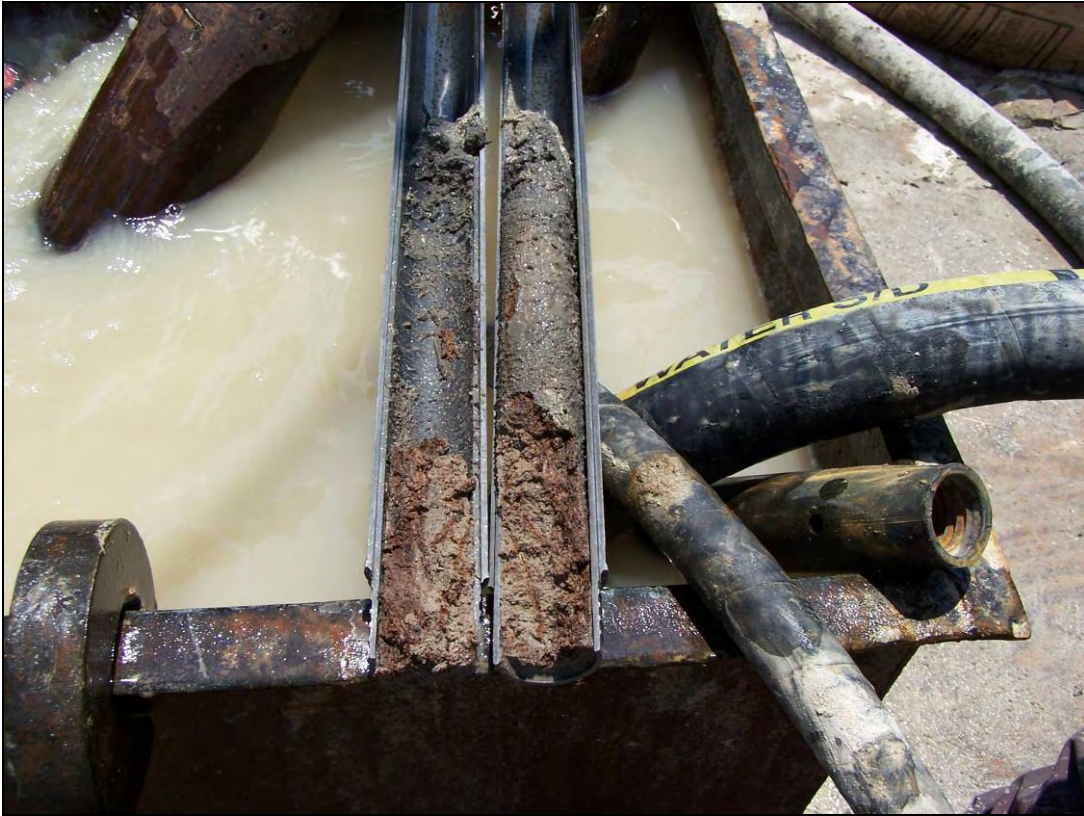
Split spoon recovery from rock boring depth of 0ft to 2ft
