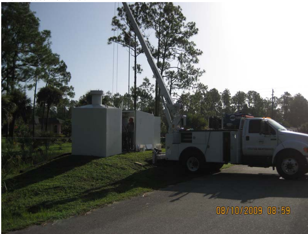
Well House Removal:
