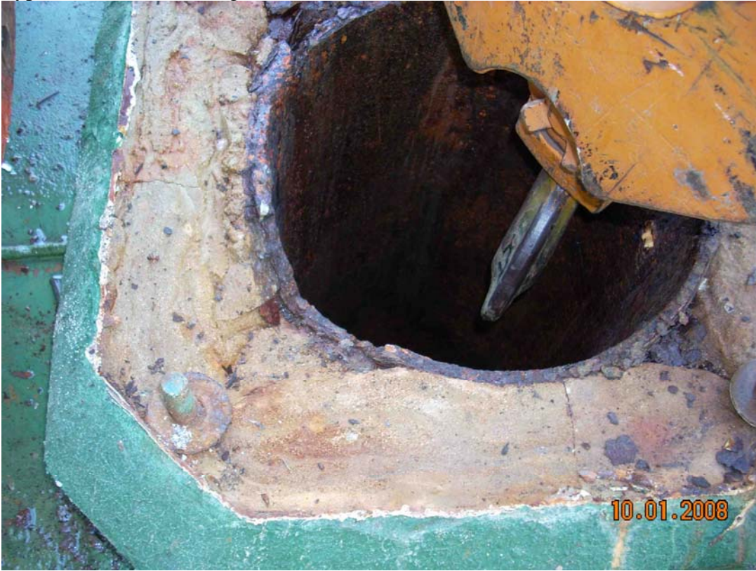
Typical Well Head Casing & Concrete Collar:
