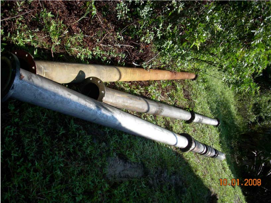
Well Piping (10' and 20' sections):
