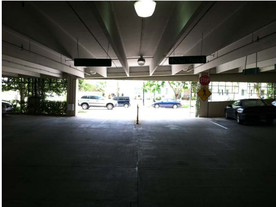
4 th Avenue South Entrance (North)
