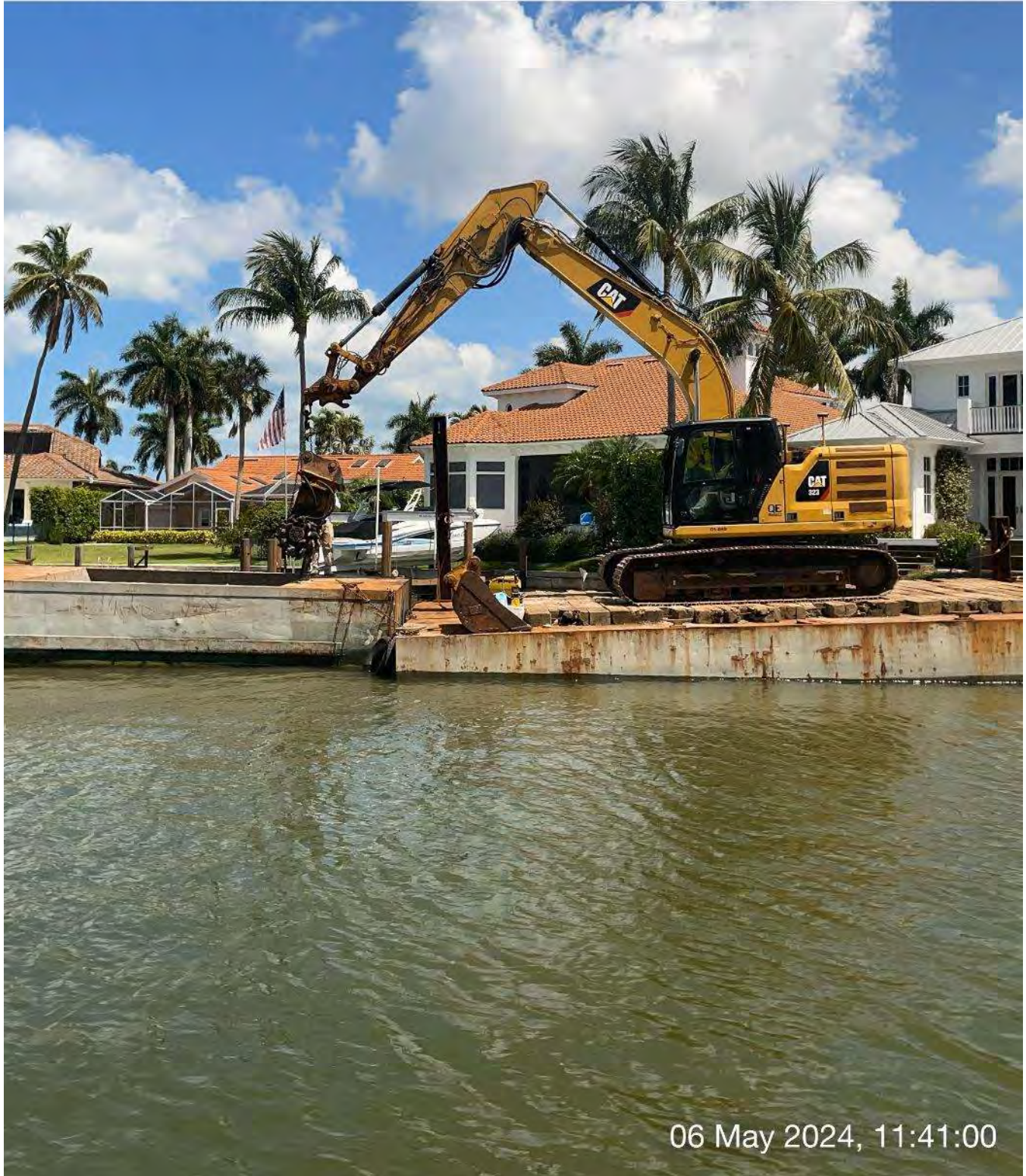
323 excavator lifting Epric grinder out of hopper.
