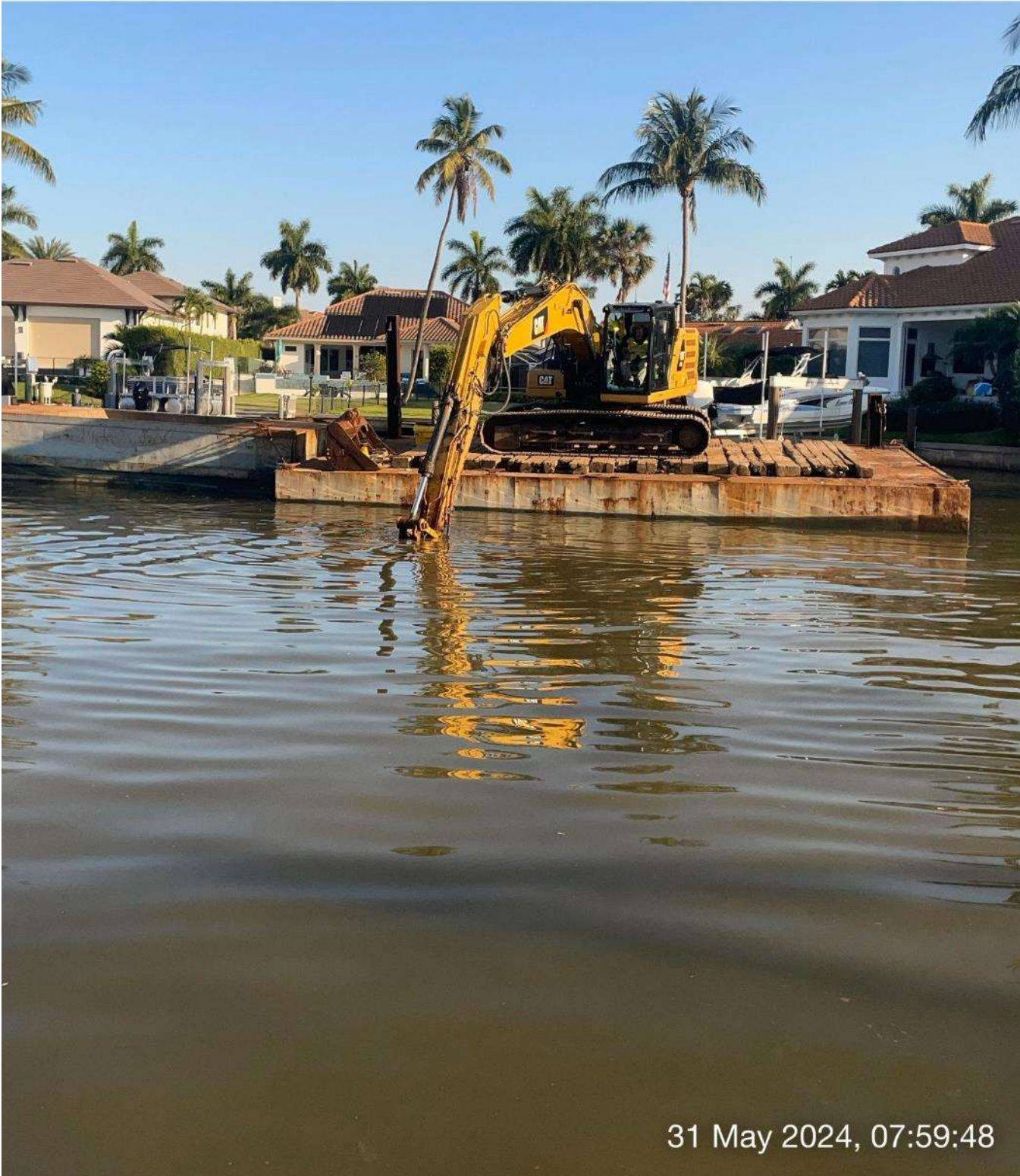
323 excavator grinding rock at station 13+20 in Canal A-A.
