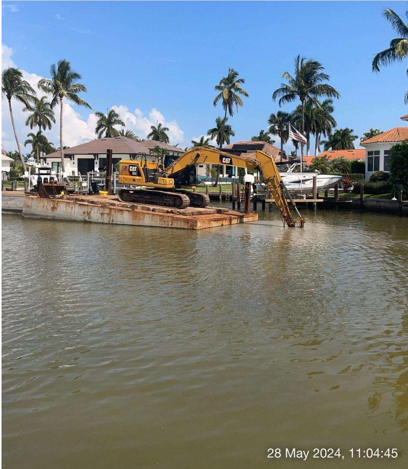
323 excavator grinding rock at station 13+60 in Canal A-A.
