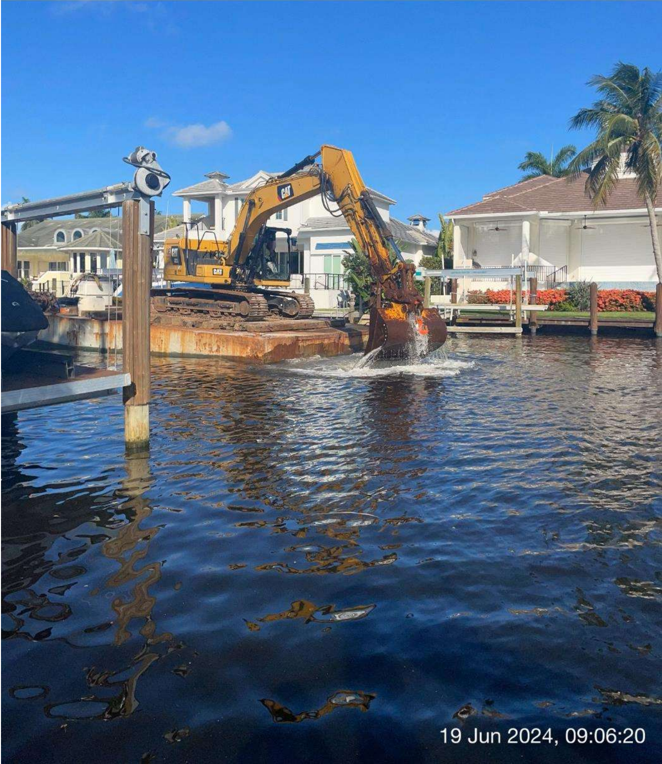
323 excavator dredging at station 8+00 in Canal A-A.
