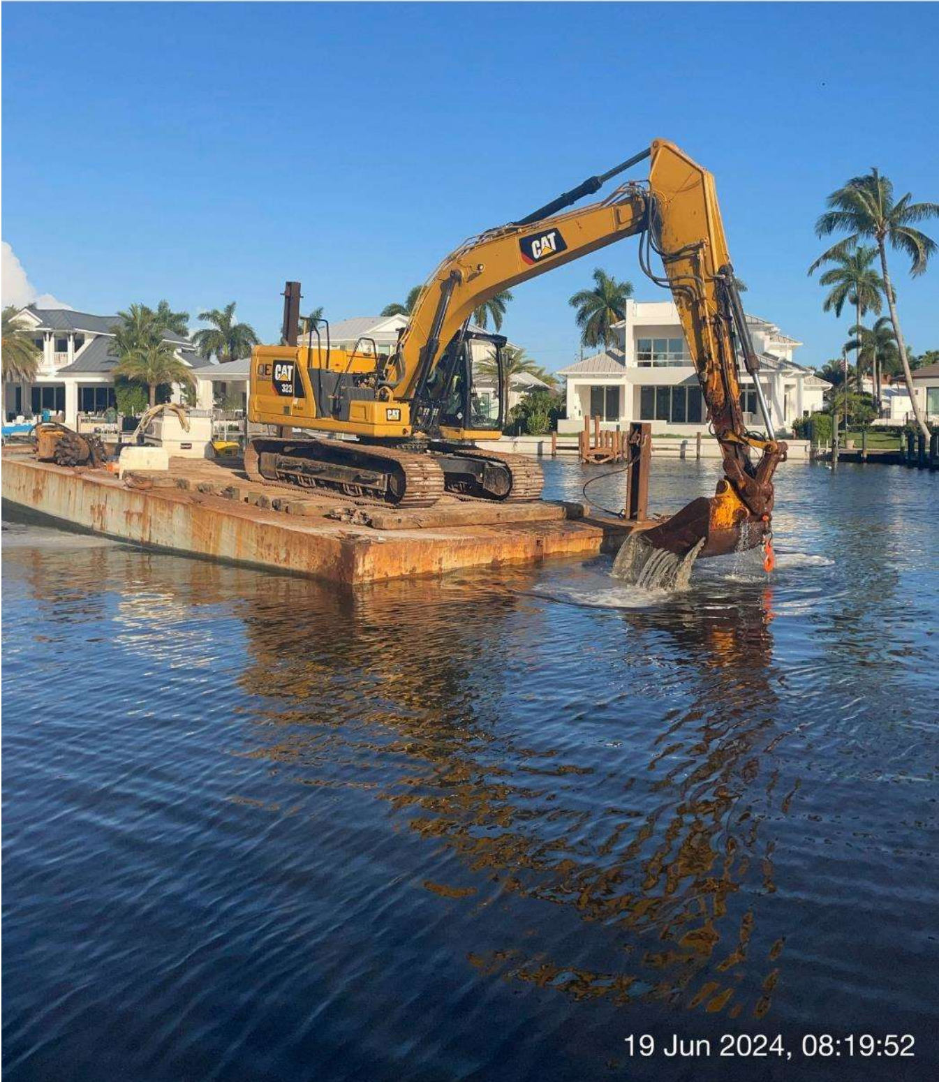
323 excavator dredging at station 12+00 in Canal A-A.
