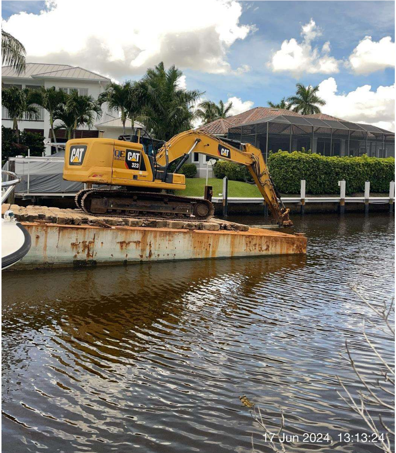
323 excavator grinding rock at station 14+50 in Canal A-A.
