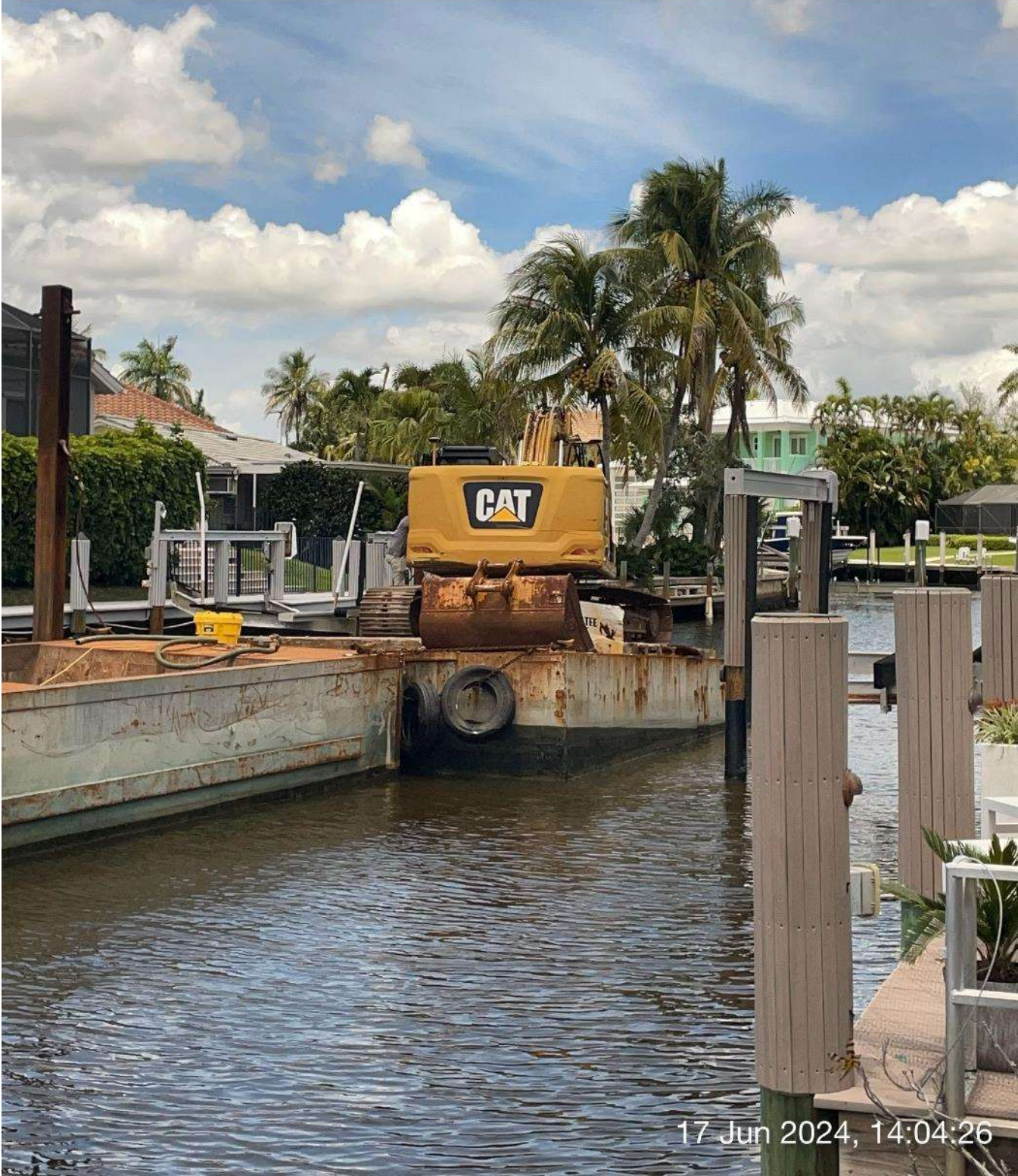
323 excavator grinding rock at station 15+00 in Canal A-A.
