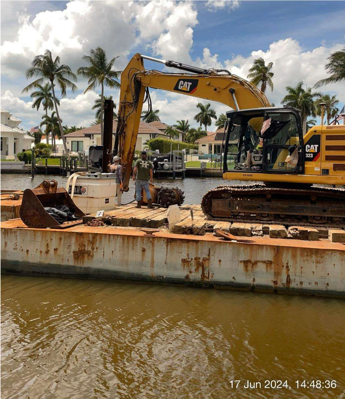
Contractor removing Epiroc grinder attachment from the 323 excavator.
