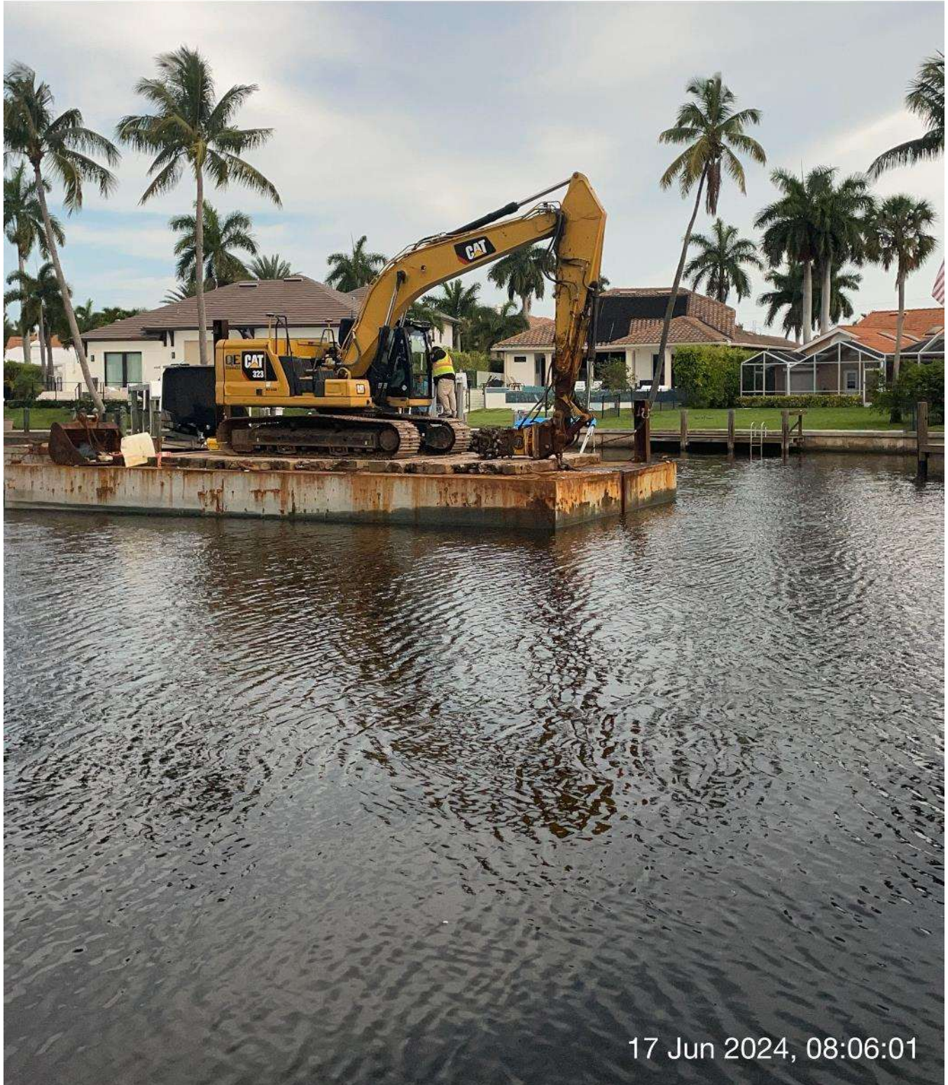
Survey crew working on 323 excavator GPS system.
