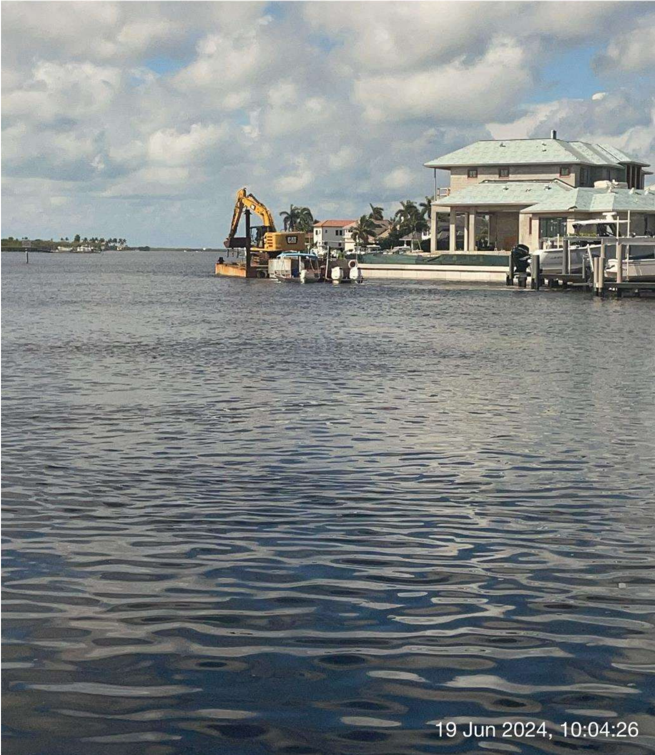
323 excavator dredging at station 0+00 in Canal A-A.
