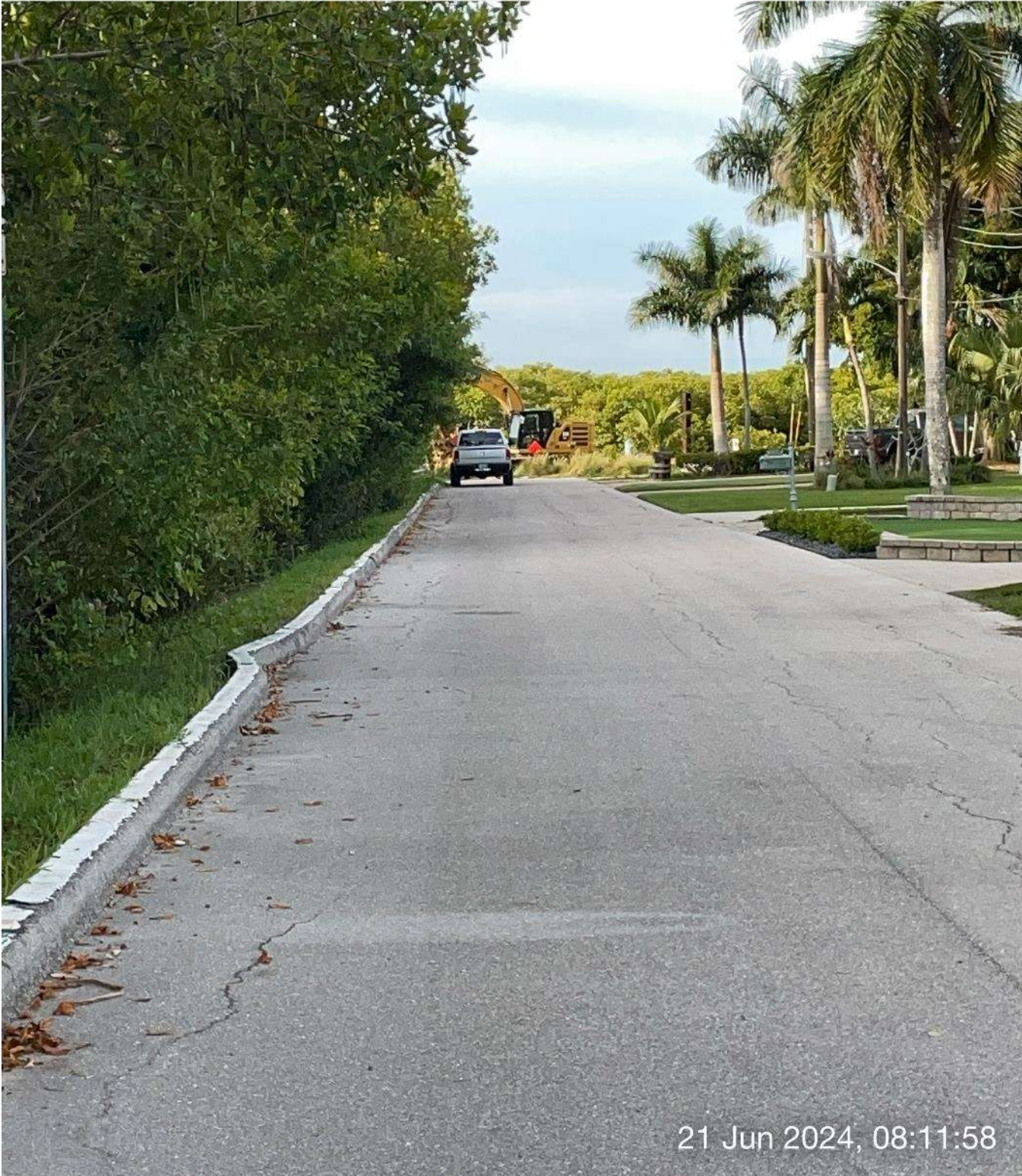
Contractor waiting on survey crew.
