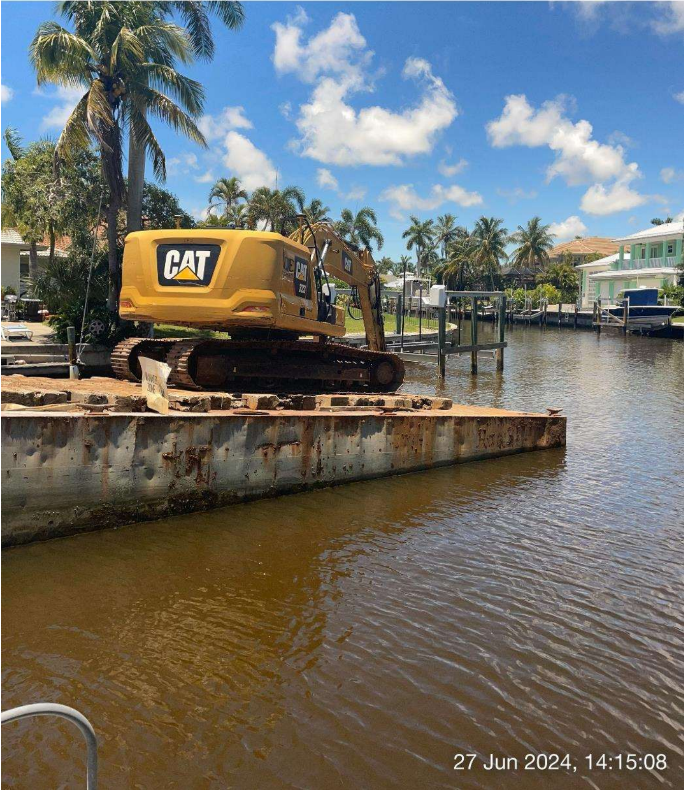
323 excavator grinding rock at station 16+00 in Canal A-A.
