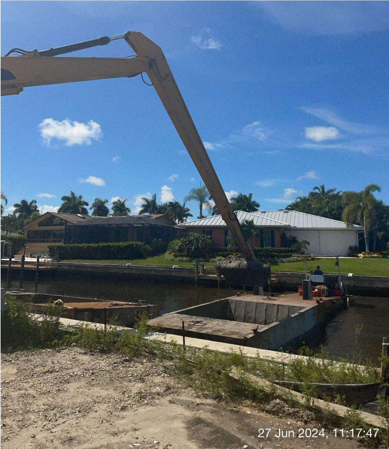
Long reach excavator removing sediment from hopper.
