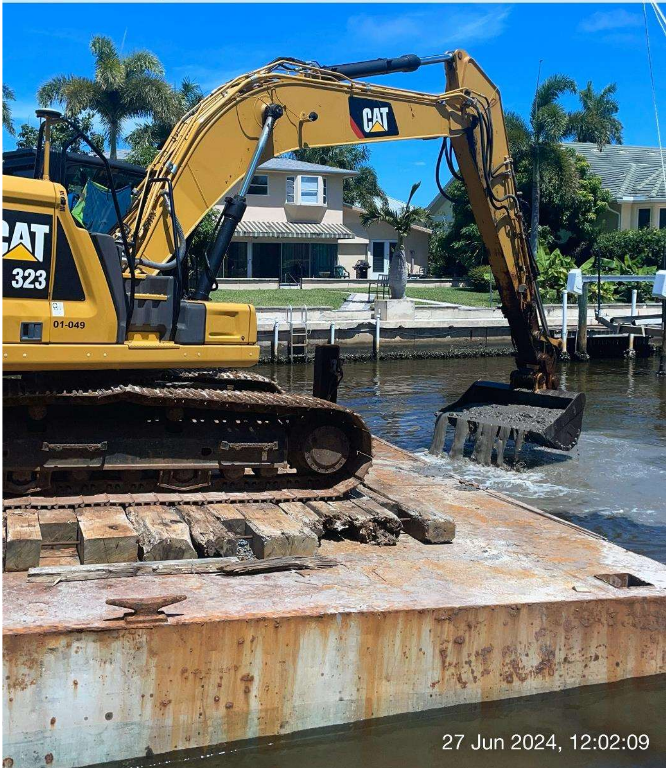
323 excavator removing sediment at station 7+00 in Canal A-A.
