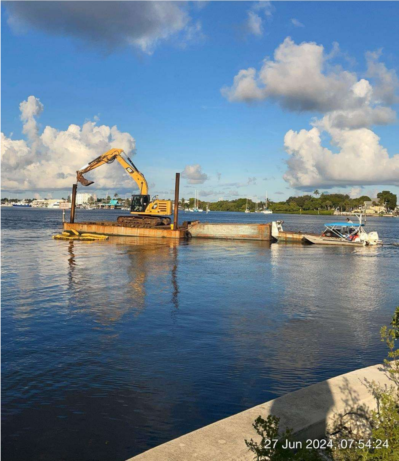
Contractor transporting equipment to Canal A-A.
