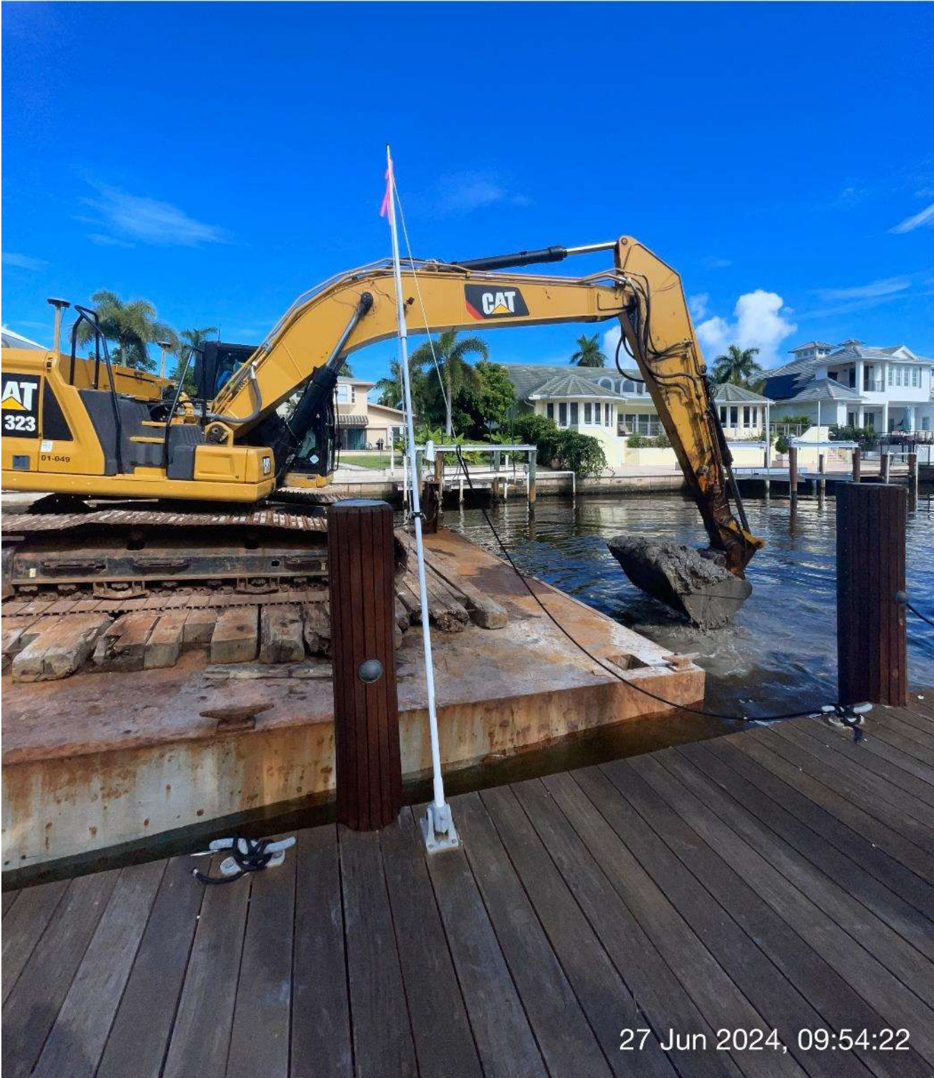
323 excavator removing sediment at station 7+50 in Canal A-A.
